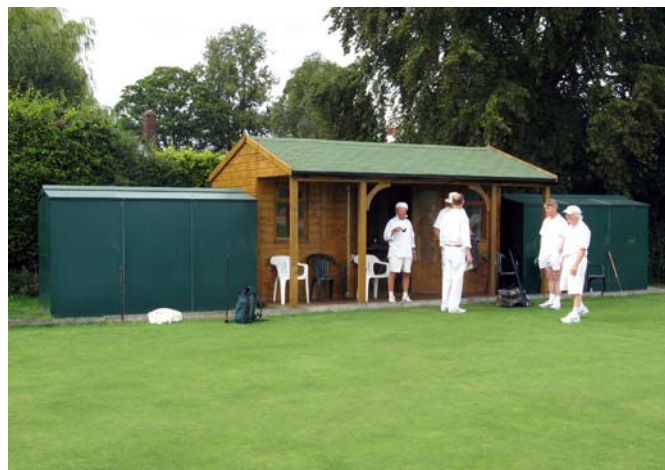
The Letchworth clubhouse and equipment sheds.
